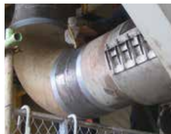
Repair to welds
