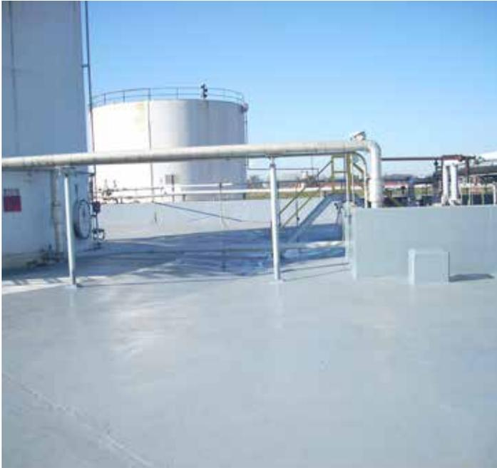
Belzona 5811 (Immersion Grade) is a solvent-free system for the protection of metallic and non-metallic surfaces operating under immersion conditions in contact with aqueous solutions.
